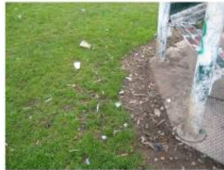
J. Rubbish around shelter
