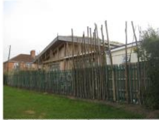
E. Innovative security fence treatment to nursery boundary
